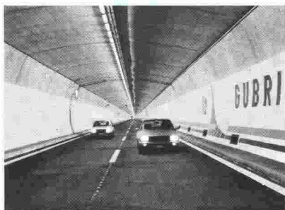
Tunnel de Gubrist, N20
