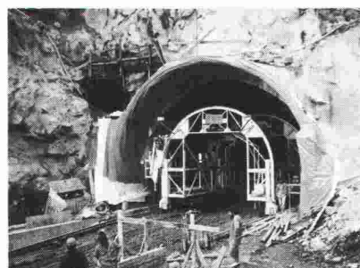
Tunnel Chûebalm, N8
