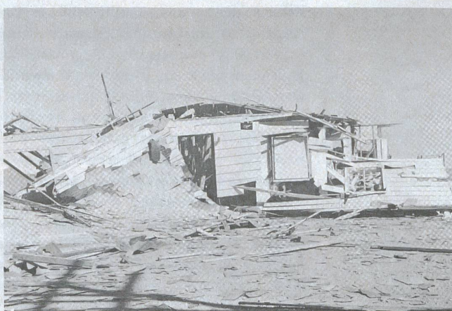
Figure 5.35. Rambler-type house after a nuclear explosion (5 psi overpressure).
