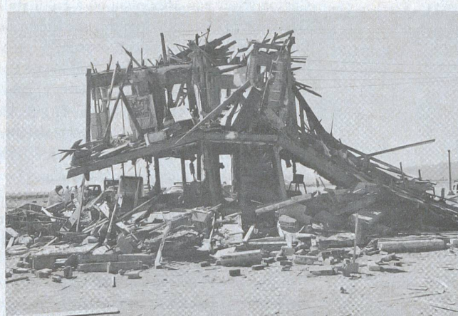
Figure 5.30. Unreinforced brick house after a nuclear explosion (5 psi over pressure).
