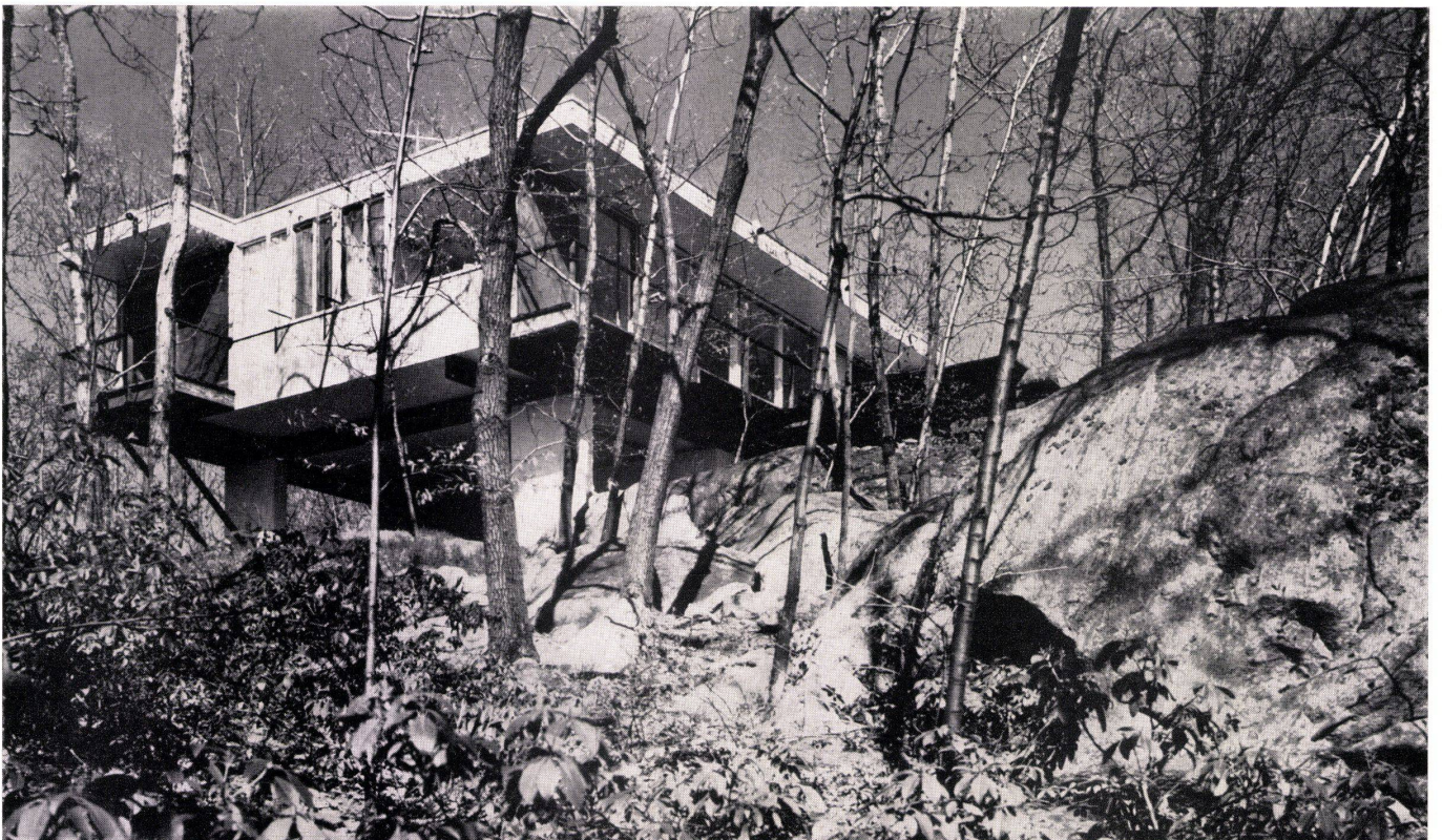
Blick von Westen. Vue de l'ouest. View from the west.
