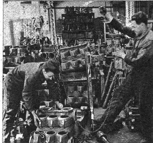
Materiallager, Transport schwerer Pumpenkörper
