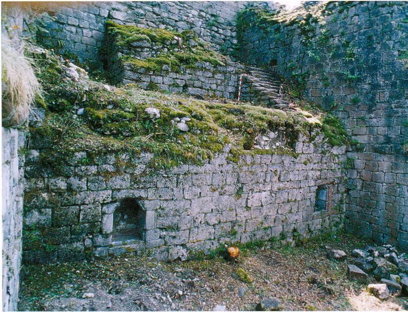
Fig. / Abb. 34 Annexes de la tour centrale (B. 26 et 27) Anbauten des zentralen Turms (B. 26 u. 27)
