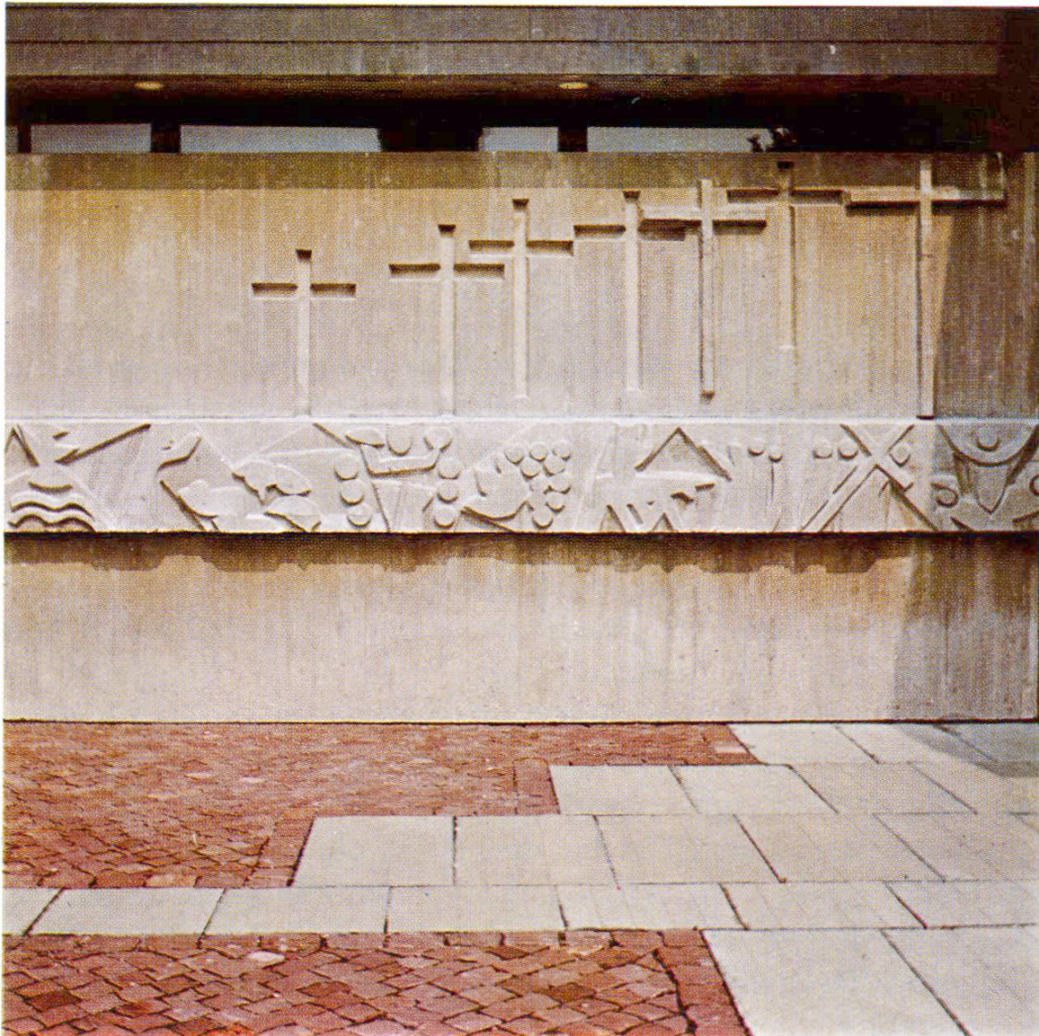
Detail des Beton-Reliefs
