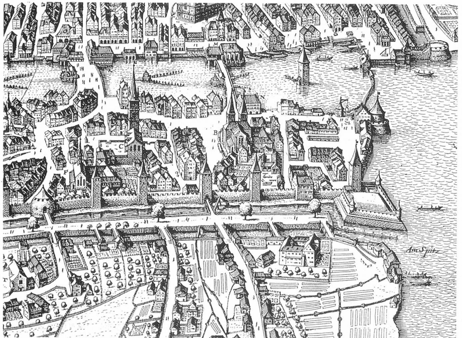
District of Paradeplatz in 1640 (SOGENAL)
