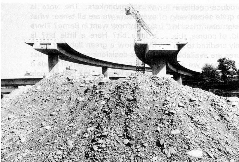
Fair shares for road and rail: building a motorway in Basle
