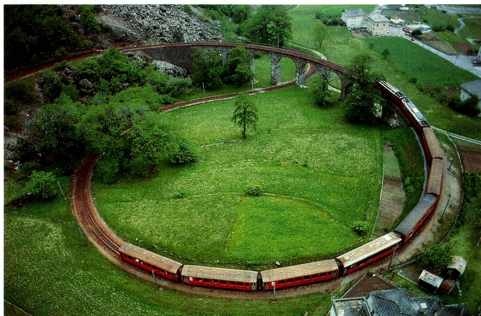
Circular viaduct to overcome the steep gradient near Brusio in the Poschiavo region.
