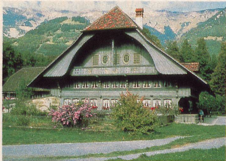
Multi-purpose house from Ostermundigen, Canton of Berne, 1797. Solid farmhouse built by Lieutenant-Captain Bendicht Gosteli. (archive photo)
