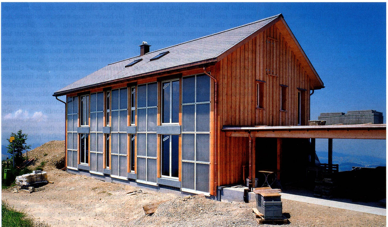
A pilot project in Canton Appenzell: the new technology of transparent heat insulation turns house walls into suppliers of solar energy. (Photo: Oerlikon Journalisten)
