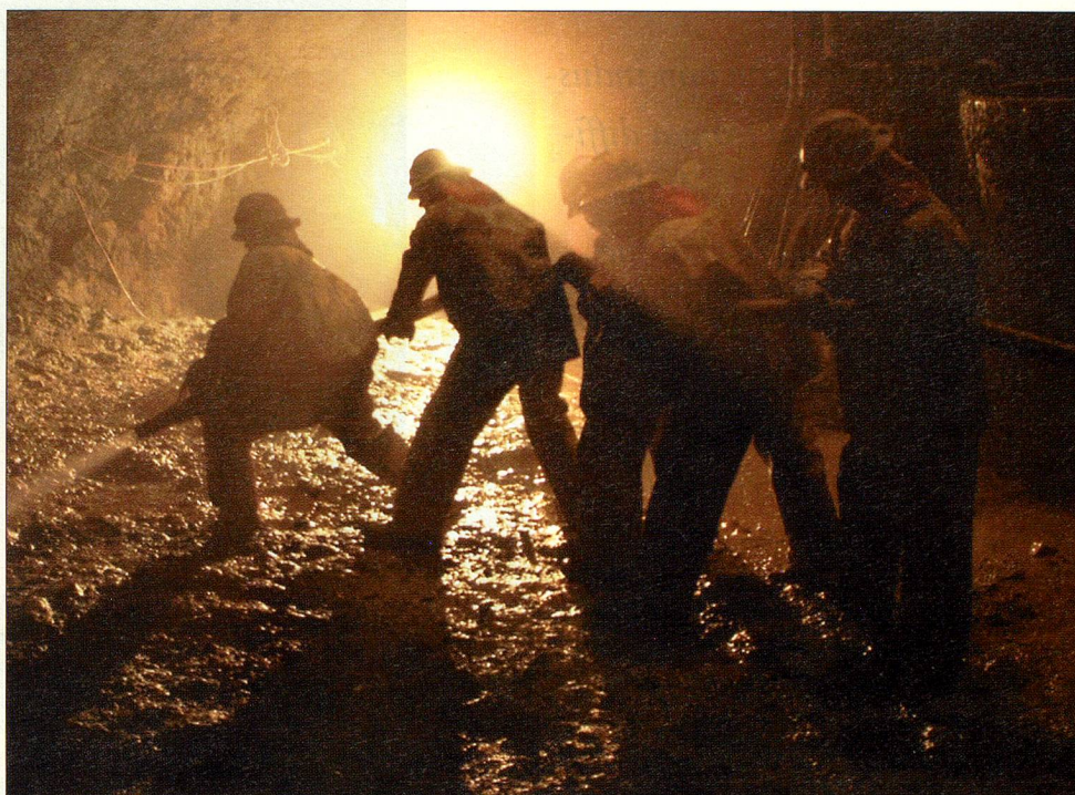
Teamwork is a must for underground construction.
