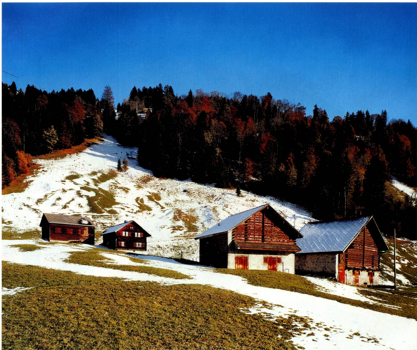
Stalls and house, artillery bunker, Ennetberg GL: The bunker on the left dates from 1979, the bunker on the right from 1980. The photographs are taken from «Falsche Chalets» («Faux chalets») by photographer Christian Schwager (Edition Patrick Frey)
