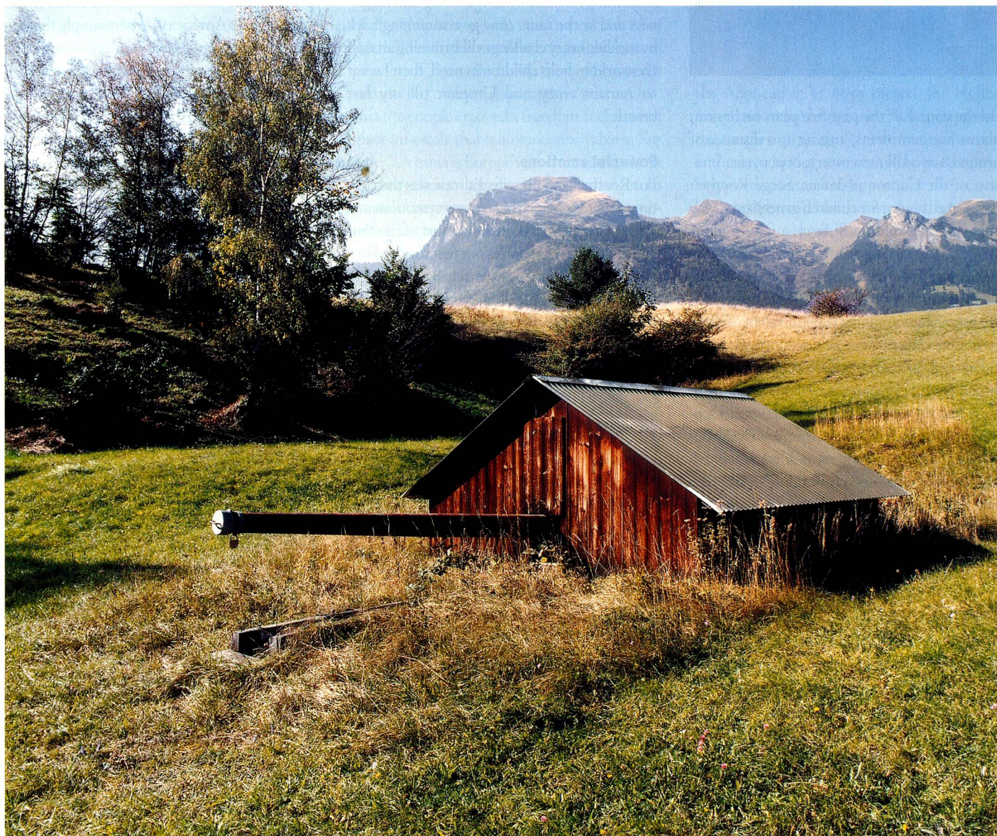
Hut, 1939–43, armoured turret of the Magletsch fortress, Oberschan SG: The turret is covered with planking and a corrugated metal roof. The tank gun barrel is not camouflaged and the mouth is covered.
