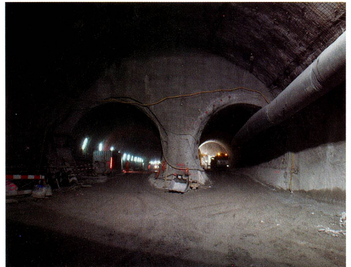
At 57 kilometres, the new base tunnel is the longest railway tunnel in the world.
