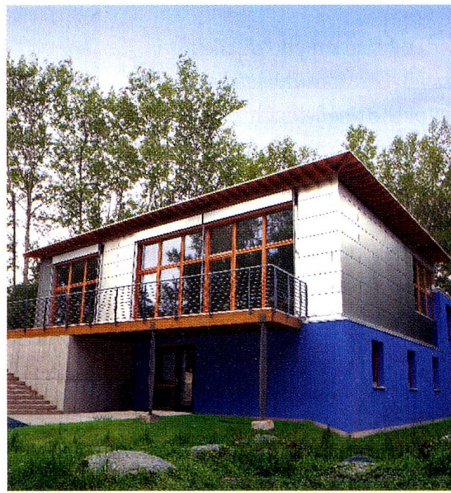
Main exterior view of first certified Passivhaus in North America: Waldsee BioHaus.
