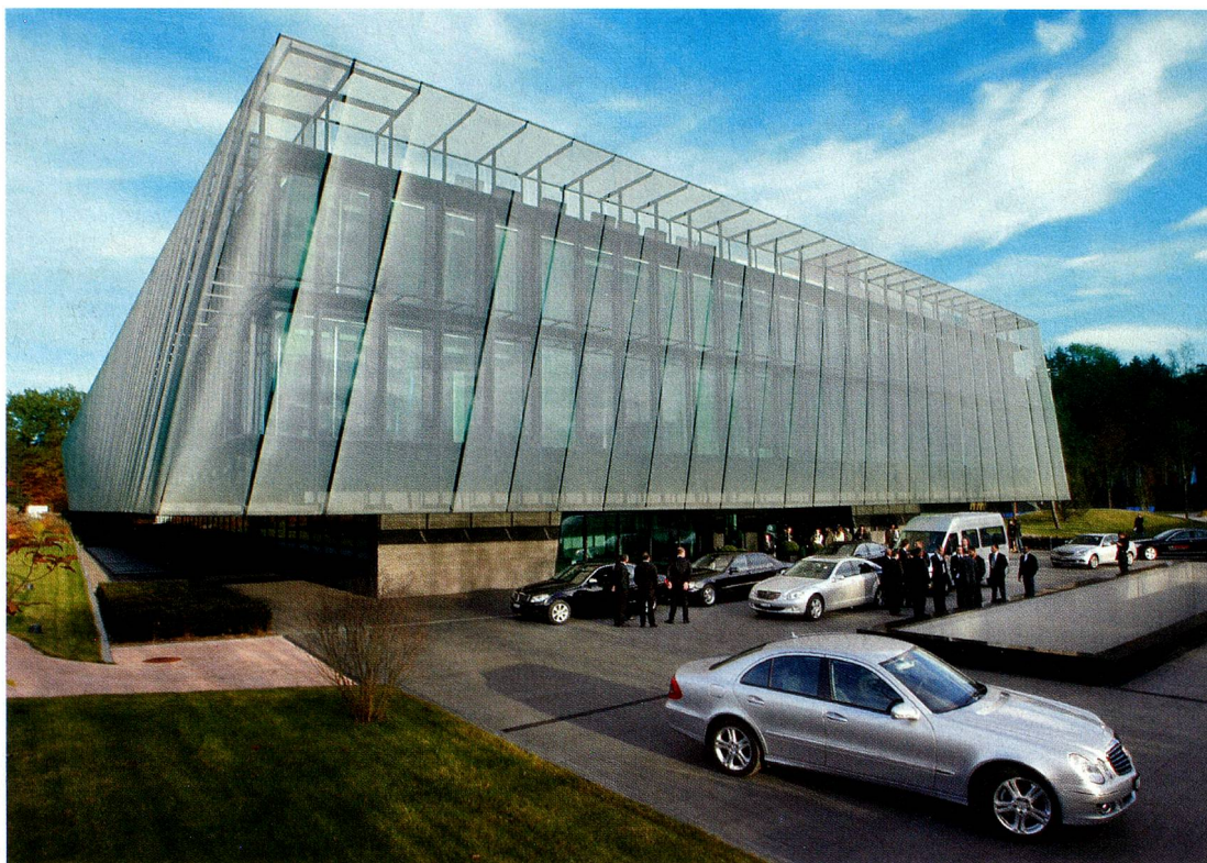
Special entrance for officials at FIFA's headquarters in Zurich
