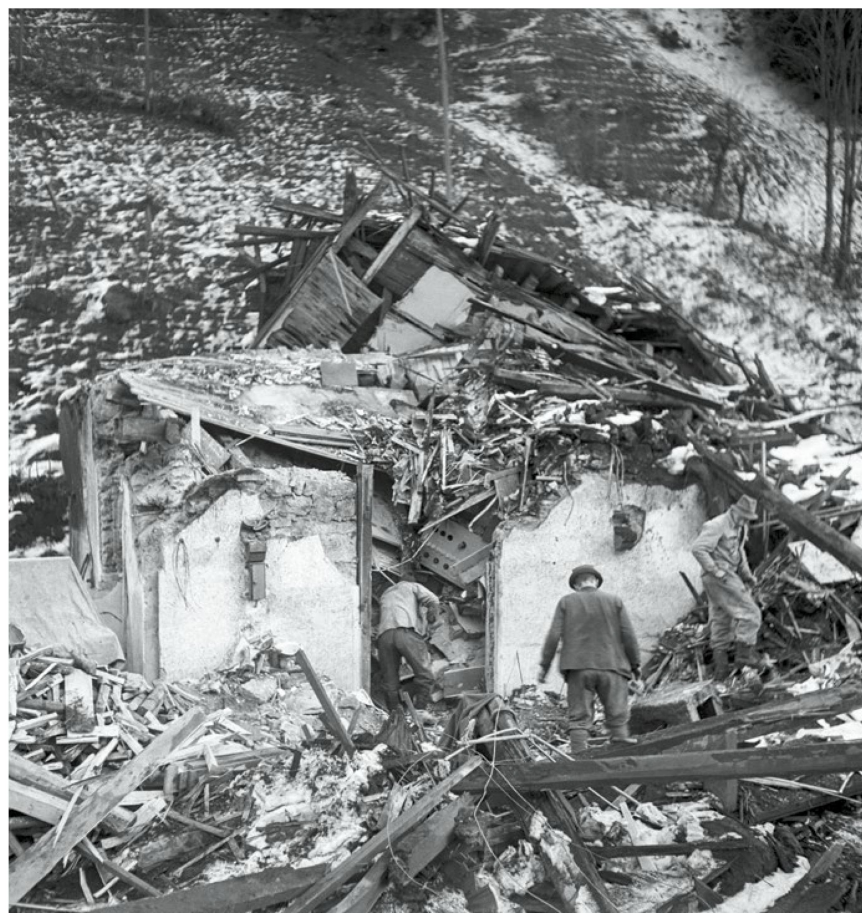
Debris in the village after the 1947 explosions – nine people died and many houses were destroyed.
