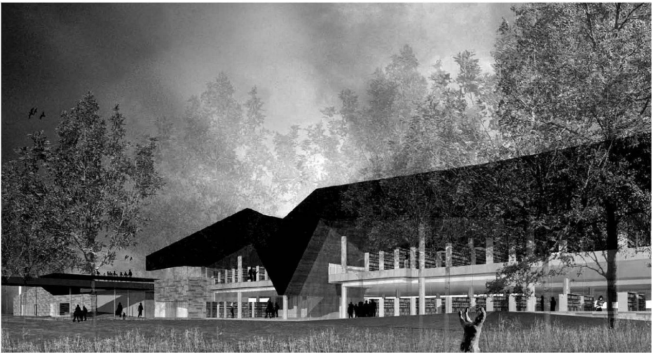
Fig. 2: View of the winning project for the Saint-Laurent library competition (Canada, 2009). Team: Cardinal Hardy/Labonté Marcil/Éric Pelletier Architectes en consortium/Leroux Beaudoin Hurens et associés inc./SDK et associés inc.
