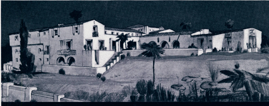
Built-in conduit and nineteen outlets provide for telephone convenience in this residence at 282 South Mapleton Drive, Holmby Hills, Los Angeles, Cal. NATIONAL THRIFT CORPORATION OF AMERICA, Builder. L. G. SCHERER, Architect, Los Angeles.
