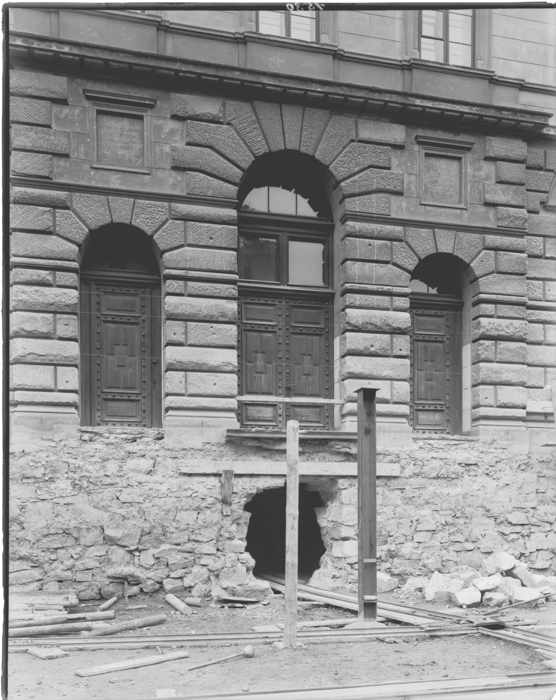
11 Gottfried Semper, Polytechnikum, Zurich; photograph of the fundamentals of the east facade during renovation, ca. 1920; Bequest of Gustav Gull, gta Archives, ETH Zurich.
