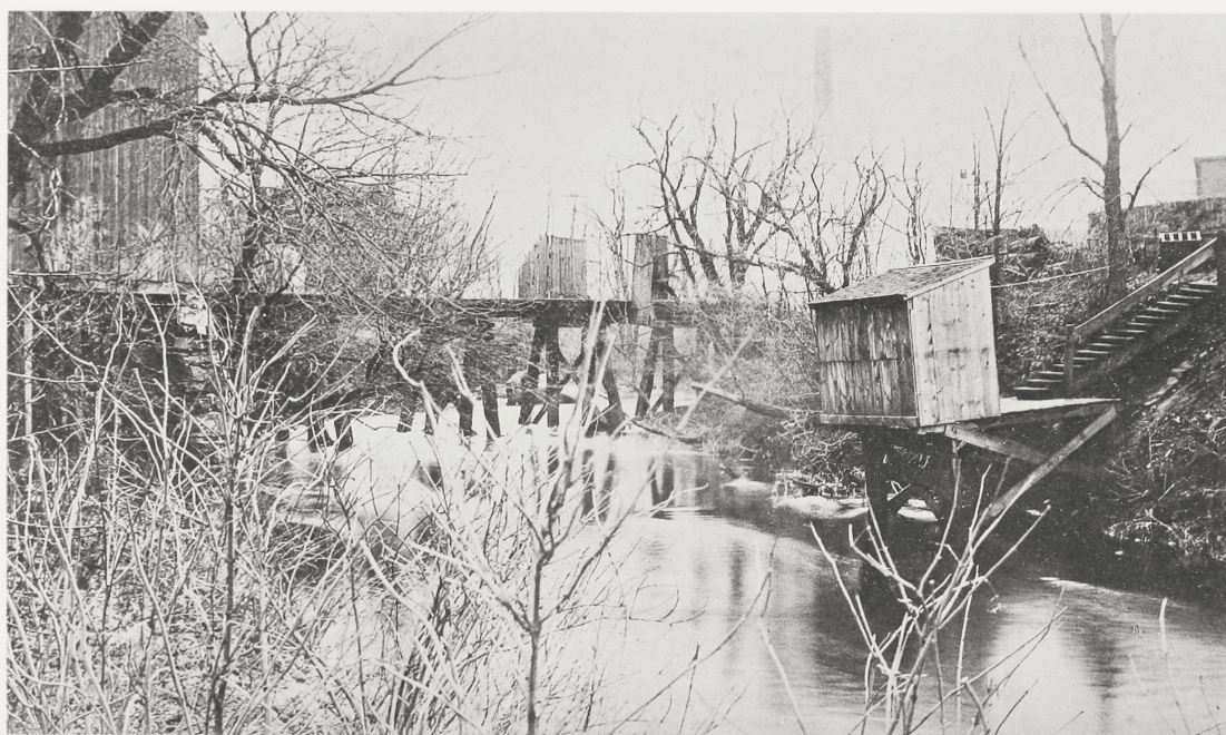
Fig. B. Privy of Foundry, overhanging Stony Brook, North Chelmsford, a Feeder of the Water Supply of Lowell. Point of Infection by T. L., (Case No. IV.)
