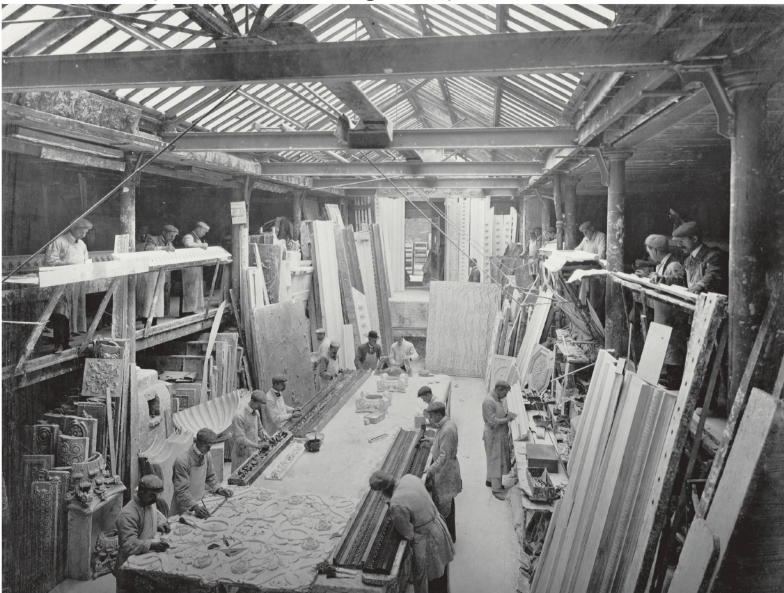
fig. 5 Workshops of George Jackson and Sons, n.d. (latter half of the nineteenth century). Workshop with fibrous plaster cornice lengths Photographer: unknown Source: George Jackson Ltd., Company Archives
