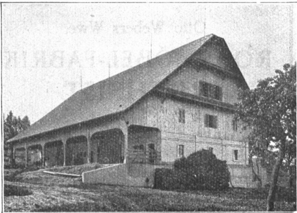
Scheune in Menznau
