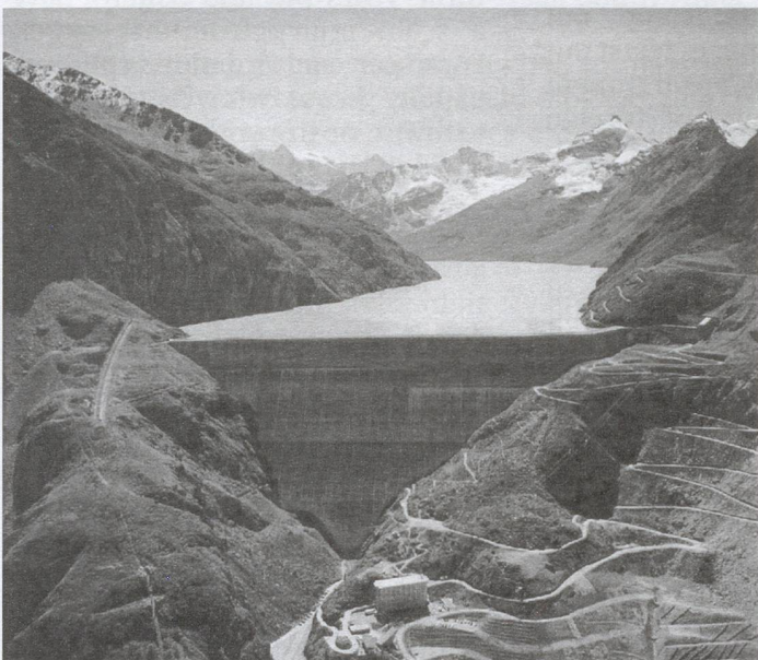
Grande Dixence dam
