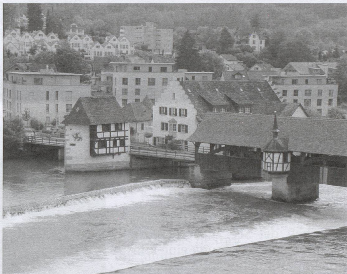
Old bridge in Bremgarten
