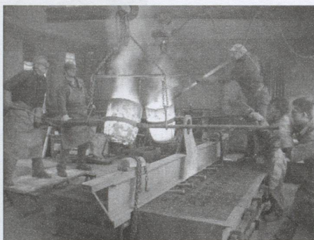
Workers in the foundry at Rüetschi AG
