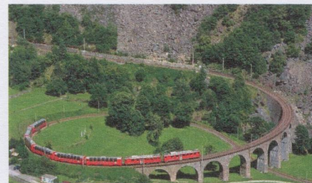
Viaduct in Brusio
