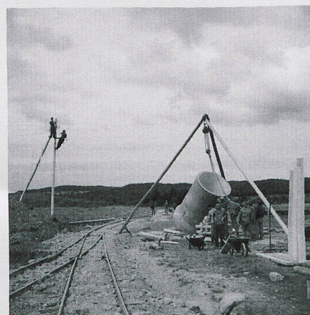
Installing large pipe to collect water, 1946
