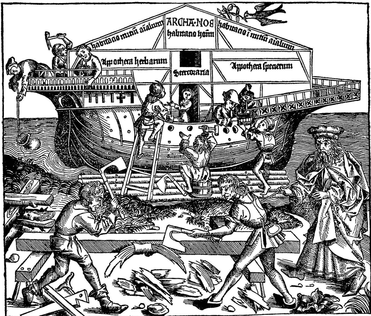
Abb. 4. Bau der Arche Noe
