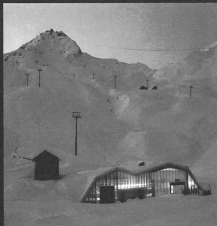
Bearth & Deplazes: Carmenna-Sesslenban, Talstation.
