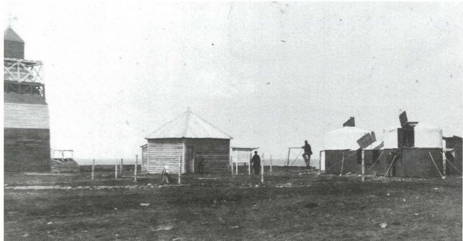
Fig. 7. Photograph of the German station in Punta Arenas. Left, wooden lighthouse of Punta Arenas, center, «tea house» and meteorological station, right, two observing domes made from iron and canvas (Archiv, Berlin-Brandenburgische Akademie der Wissenschaften).
