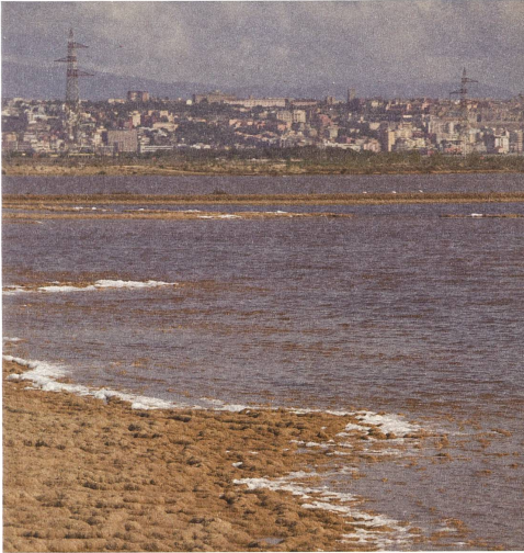
The circulation of water along the shore has been interrupted by industrial infrastructure, which creates pollution along the beach.
