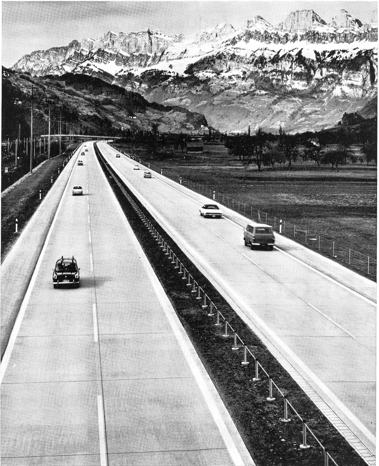
Nationalstrasse N3 Zürich-Chur, Flums-Mels, Betonbelag
