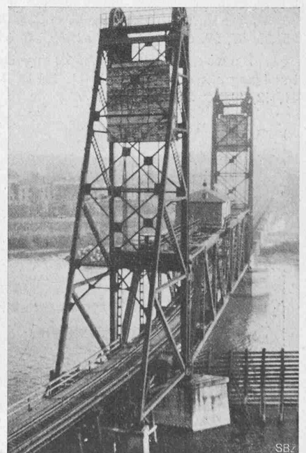
Abb. 65. Mississippi-Hubbrücke in St. Paul (Minn.).
