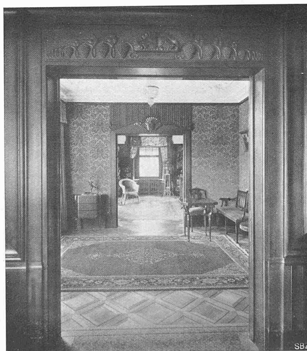
VILLA ARBENZ IN ZÜRICH 8
