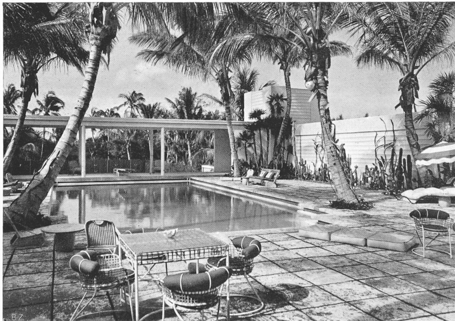
BARCLAY DOUGLAS HOUSE IN PALM BEACH, FLORIDA Arch. MAURICE FATIO, G. E. P., in West Palm Beach
