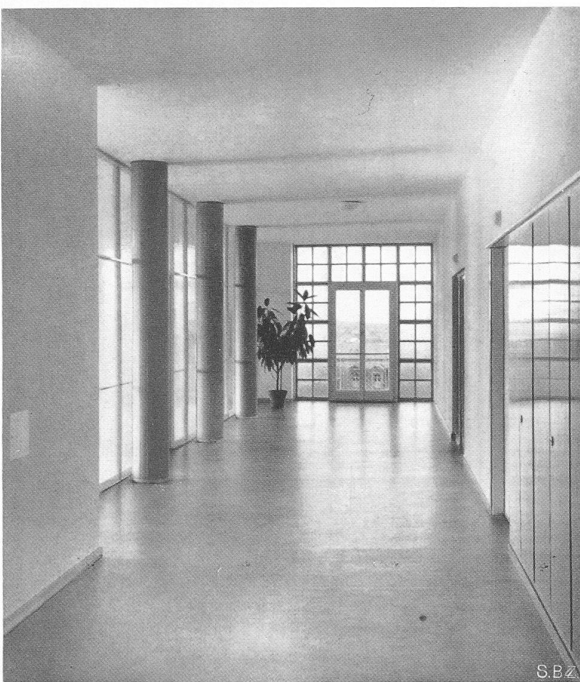
Korridor-Ende, links Tagraum
