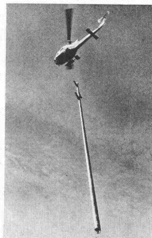
Transport eines 26-m-Mastes
