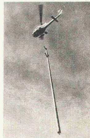
Transport eines 26-m-Mastes
