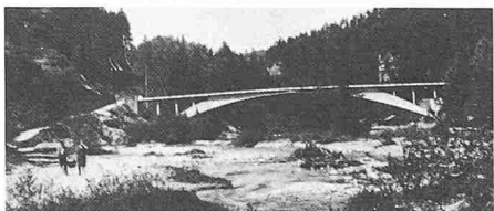
2051 Schwarzenburg 1932 Rossgrabenbrücke, Ing. Maillart Robert
