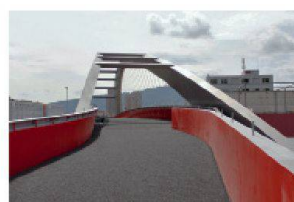
Railway overpass Zurich West huggenbergerfries Architekten Zurich
