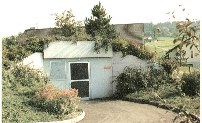
Hangeinbau-Trafostation EW Gossau
