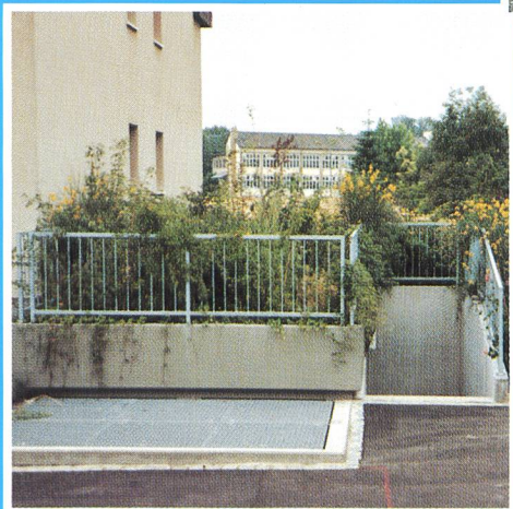
Station souterraine Unterflurstation in Sisseln/AG
