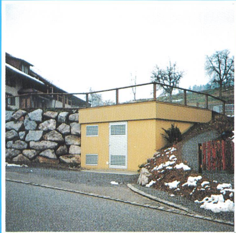
Station en talus Hangeinbaustation in Gossau/ZH
