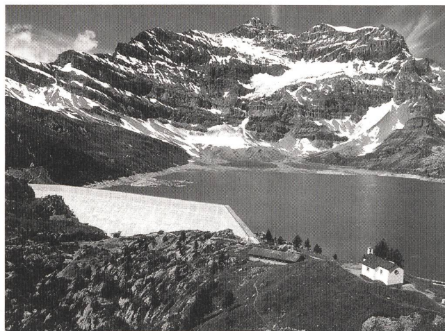
Staumauer Salanfe (VS)
