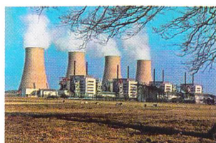
KKW Chapelcross (4x50 MW).
