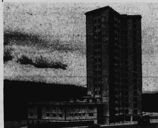
Building Les Charmettes in Frelburg, 17 Stockwerke
