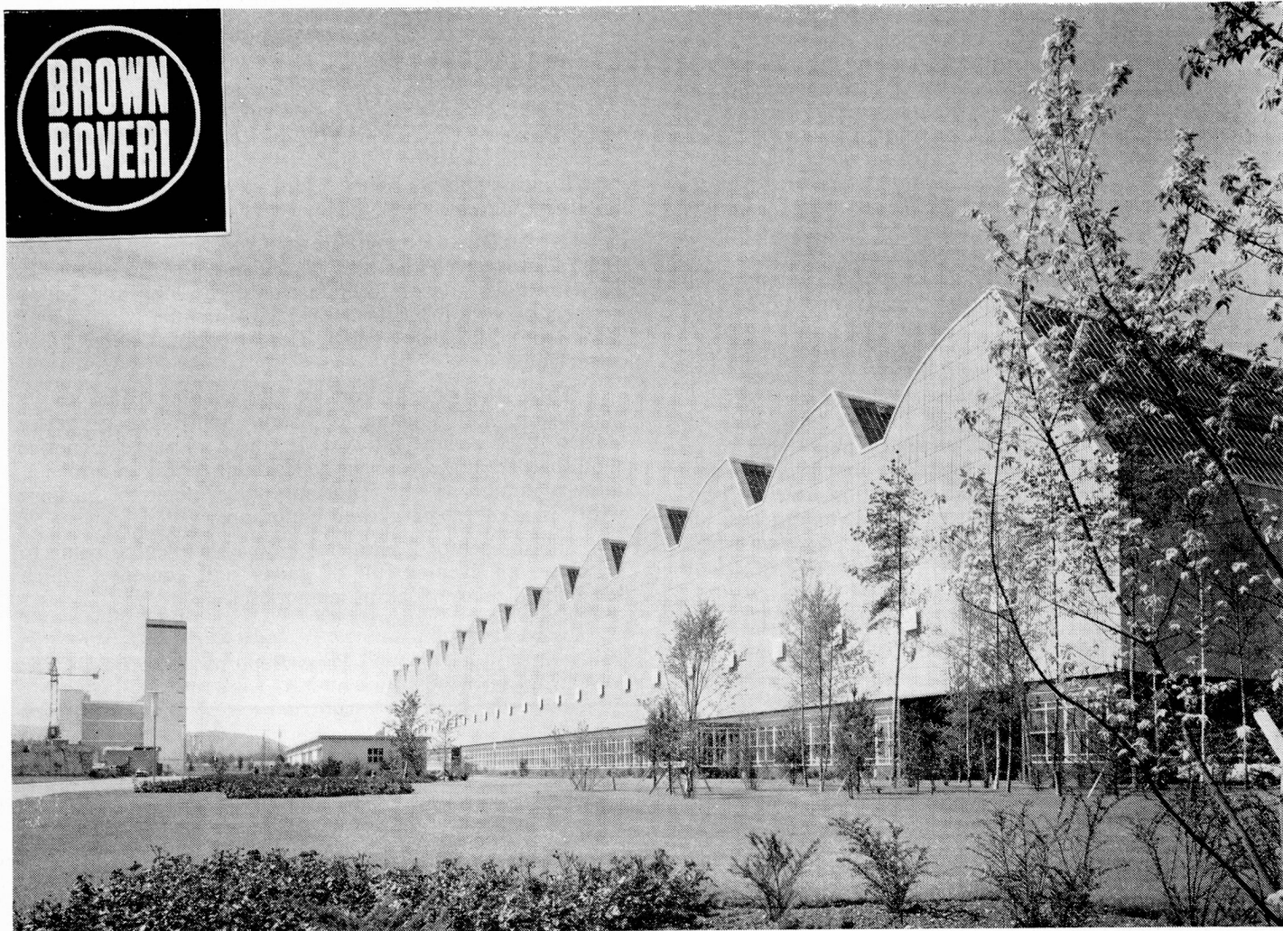
New works at Birr Aargau
