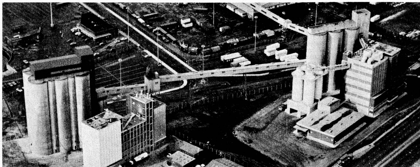
The new harbour in Seaforth, Liverpool. On the left in the foreground is Allied Mills Ltd. flour mill, 280 t/24 hours, with grain silo 17000 tons. On the right is Kellogg Co. of Great Britain, 720 t/24 hours corn mill, with 7500 t silo. Both mills were built by Bühler Brothers in 1972/73.
