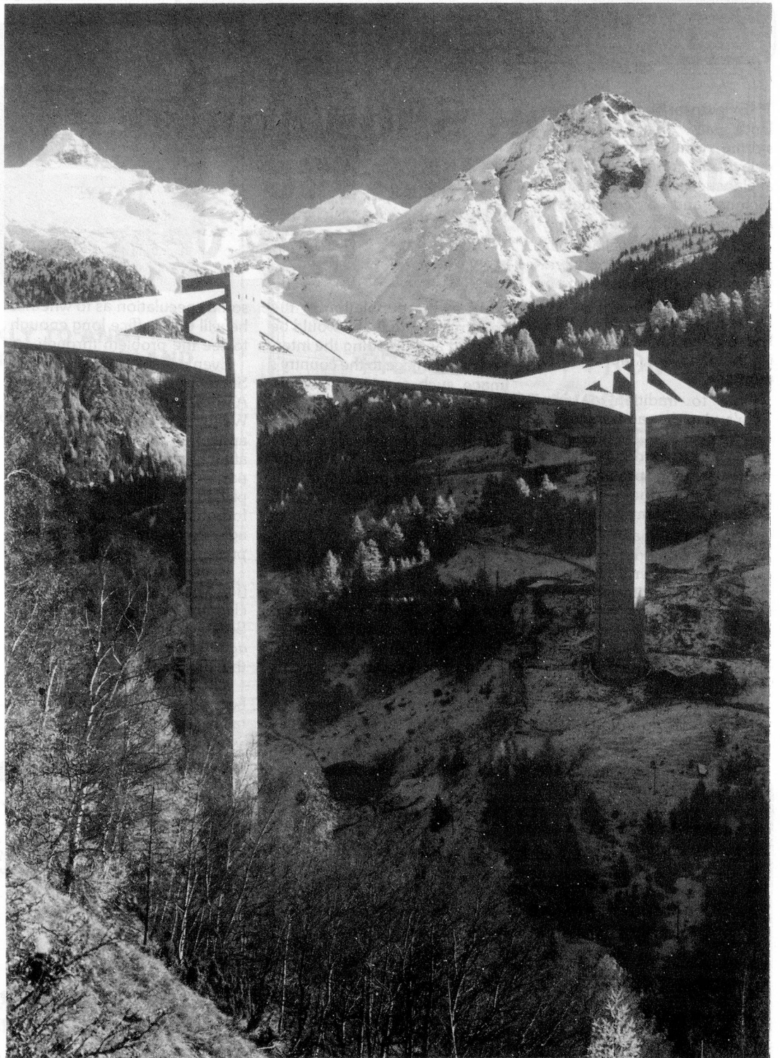
High above the Ganter, the half mile long bridge
