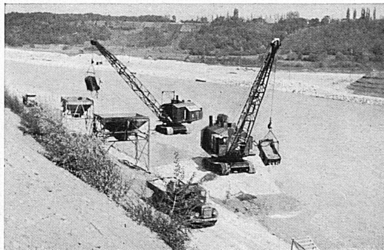
Draglines, 90 tonnes, 1 m³.
